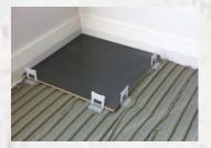
Spread your tile adhesive and lay the tile. Place LEV TEC clips underneath the tile slightly back from the edge.
